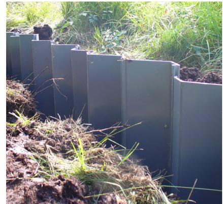
Plastic piling is the eco-friendly solution for many projects, with Liniar's high-strength, recycled pile providing developers and specifiers with an alternative to steel or timber. From sheet pile to trench pile plus the innovative log pile with timber composite fascia, the applications for Liniar piling are many and varied across a wide number of different industries. (see page 9)
